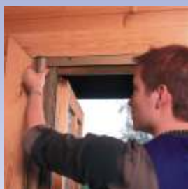
Fit the upper track into the cassette part and push it into the counterpart of the previous picture. Fasten the upper track.
